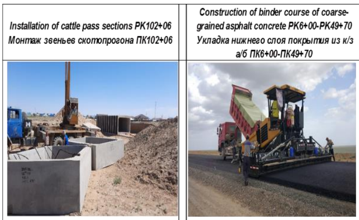
Picture 3. Road works on Lot 4: animal crossing construction and pavement works 14.06.2020
