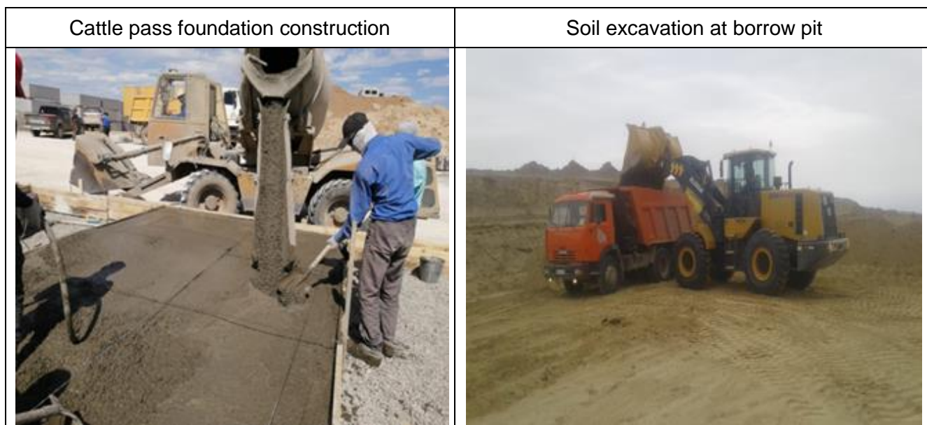
Picture 4. Lot 5 road works: foundation and excavation works, 20.06.2020
