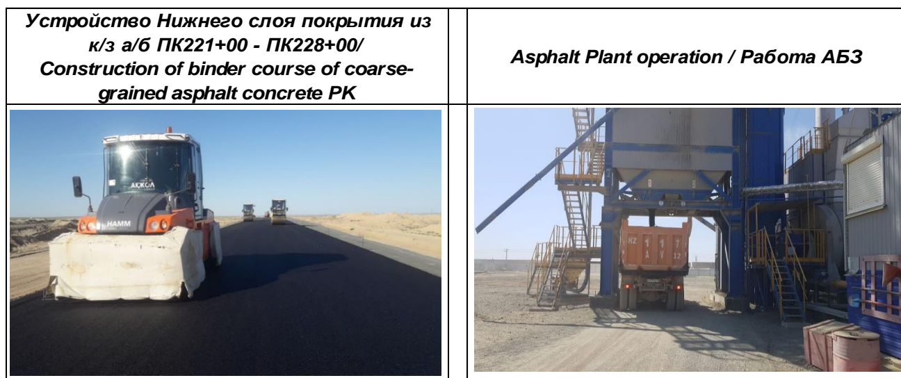
Picture 5. Lot 6 road works: asphalt laying, operation of Asphalt plant, 08.06.2020
